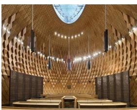
Inside the building the courtroom takes its inspiration from the seed cone of a kauri tree. The exterior of the ovoid shaped courtroom is clad in copper panels. The interior is made up of 2294 diamond shaped panels made from silver beech.
