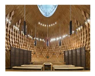
Inside the building the courtroom takes its inspiration from the seed cone of a Kauri tree. The exterior of the ovoid shaped courtroom is clad in copper panels. The interior is made up of 2294 diamond shaped panels made from silver beech.
